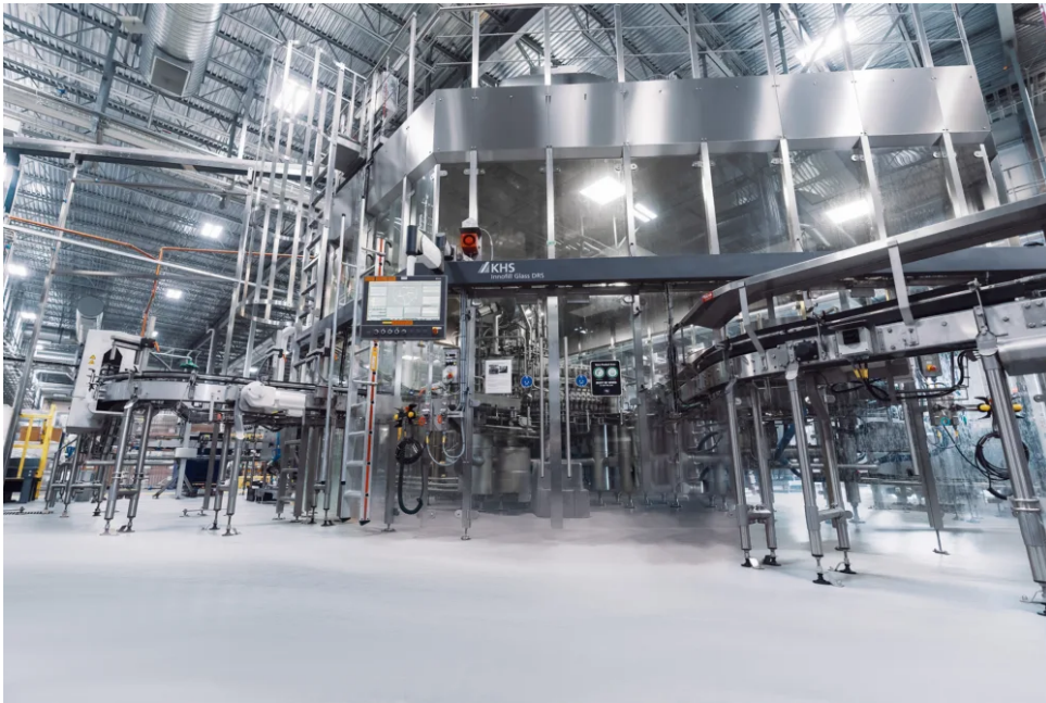
↑ Part of the KHS glass line is the Innofill Glass DRS filler that fills up to 36,000 341-milliliter bottles per hour.
