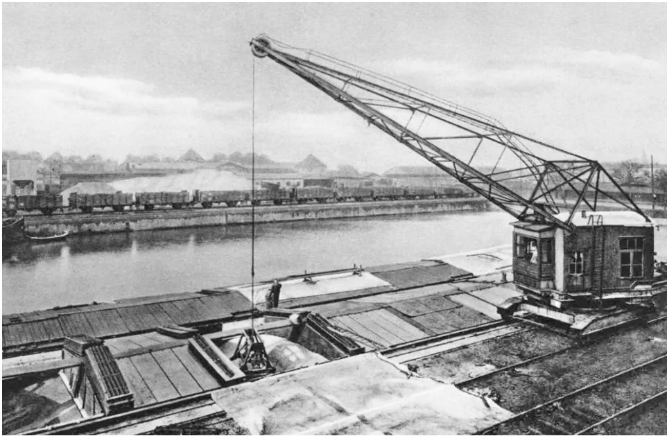
↑ Unloading brewing barley at the docks in Dortmund, opened by Emperor Wilhelm II in 1899 and now the largest canal port in Europe.
